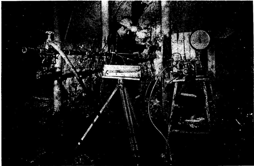
Fig. 15.- Testing a gas drainage hole under suction at West Cliff Colliery.
